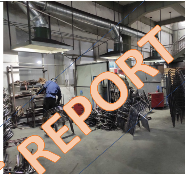
Equipment-Welding, shot blasting equipment -15 sets(1/2)
